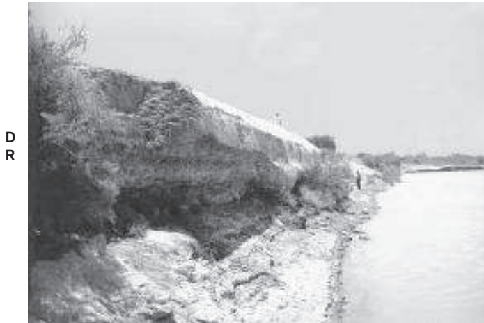
Figure 26. The oldest river retaining wall in the world in Khuzestan province.
