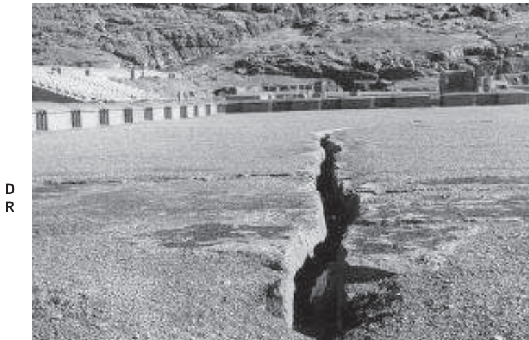
Figure 5. The general layout of the open air water ways in the Takht-Jamshid palace.
