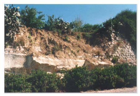
Photo 2. Even the existing regulation prevents demolishing or endangering the rubble walls increased soil erosion brings to their structural damage
