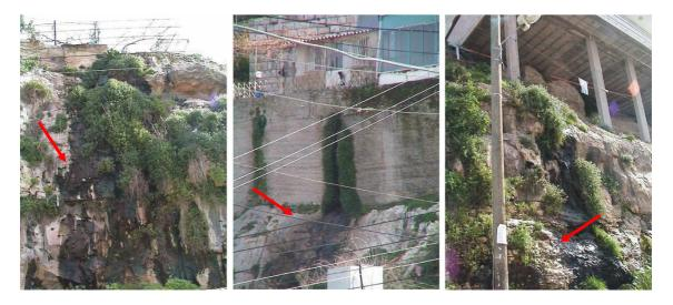
Fig. 1. Betir infected rocky surfaces due to sewage that seeps from cesspits located at higher levels (Source: Arij, 2005)
